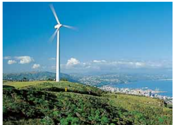
The 40 metre high Brooklyn wind turbine in Wellington.
