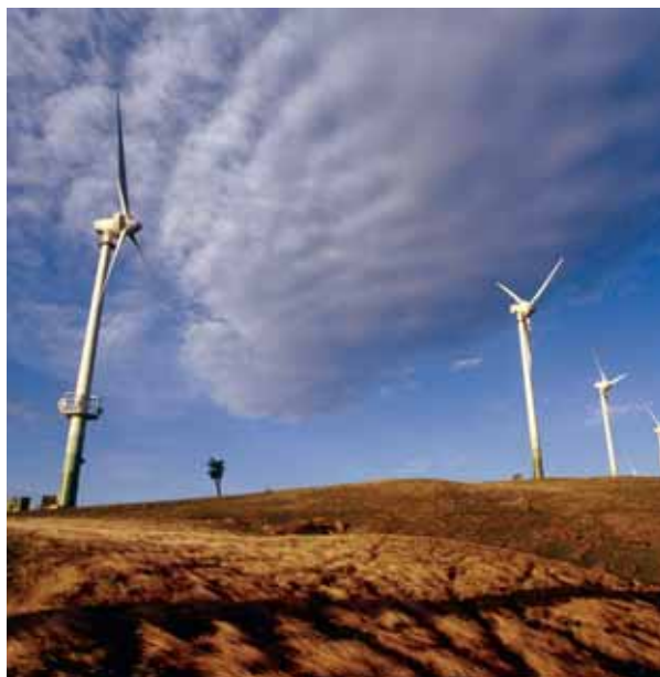
Hau Nui, a small wind farm in rural Wairarapa. Note the small transformers.
